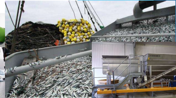
On-site compact protein processing plant.
